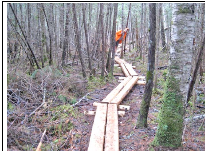
Trails through Witt Swamp are elevated where necessary to protect the underlying wetland environments.
